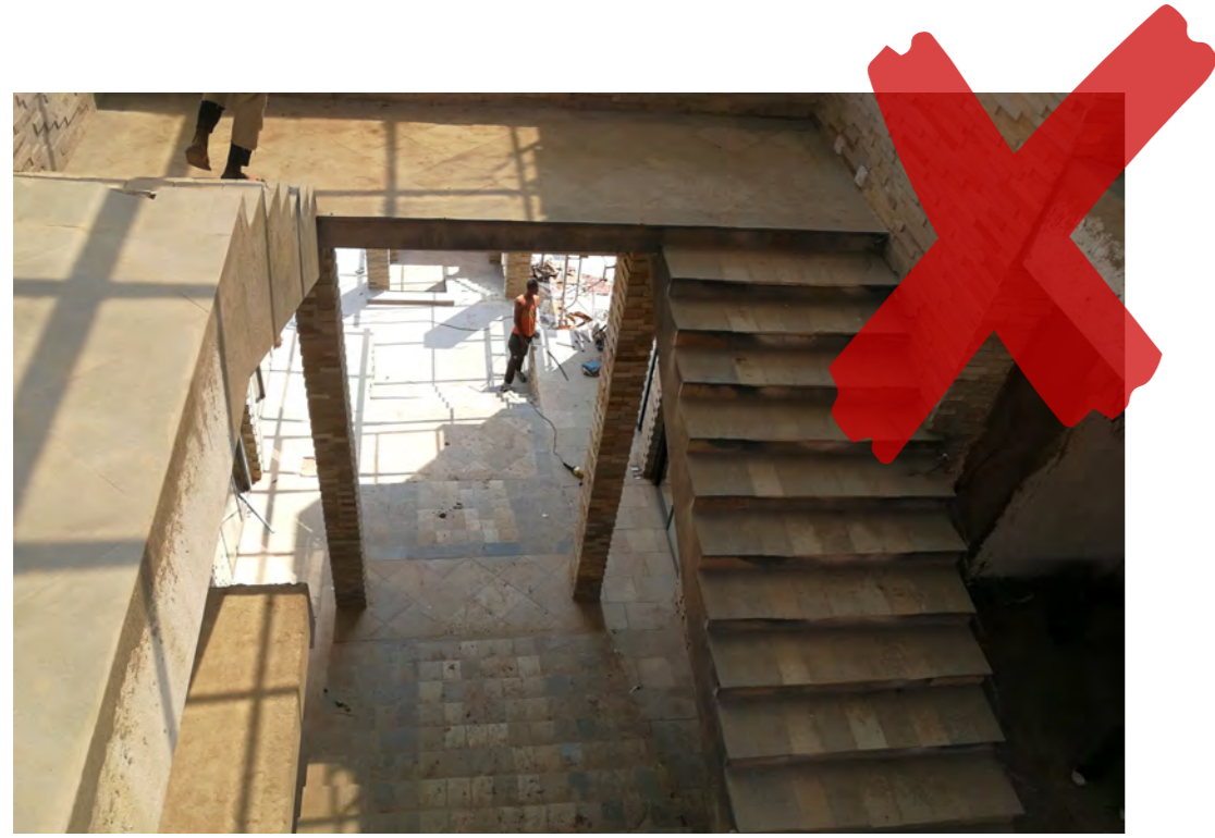
Risk of falling! Always install guard railings!
